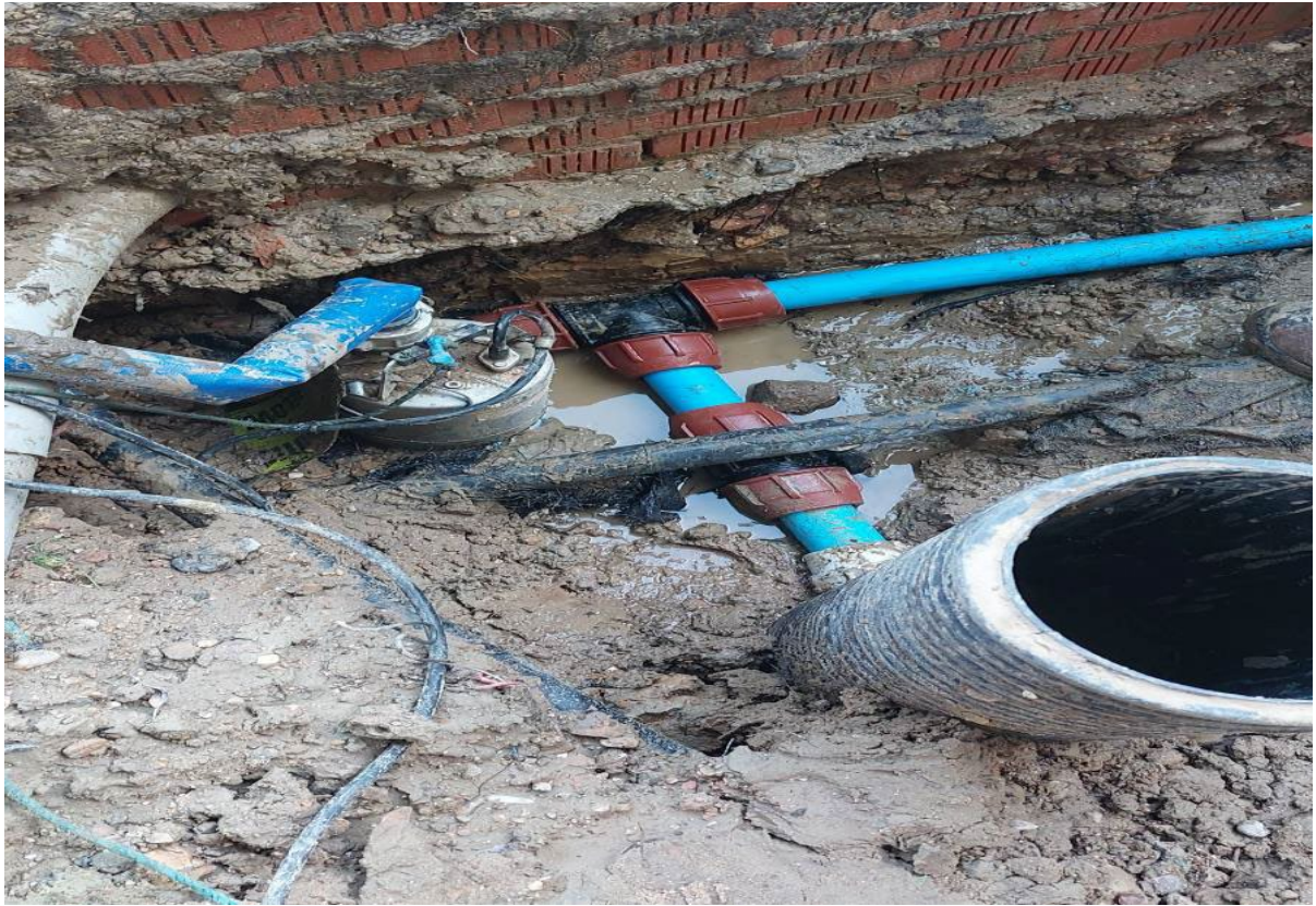
Supplied and fitted new fittings to repair the cold water supply pipe
