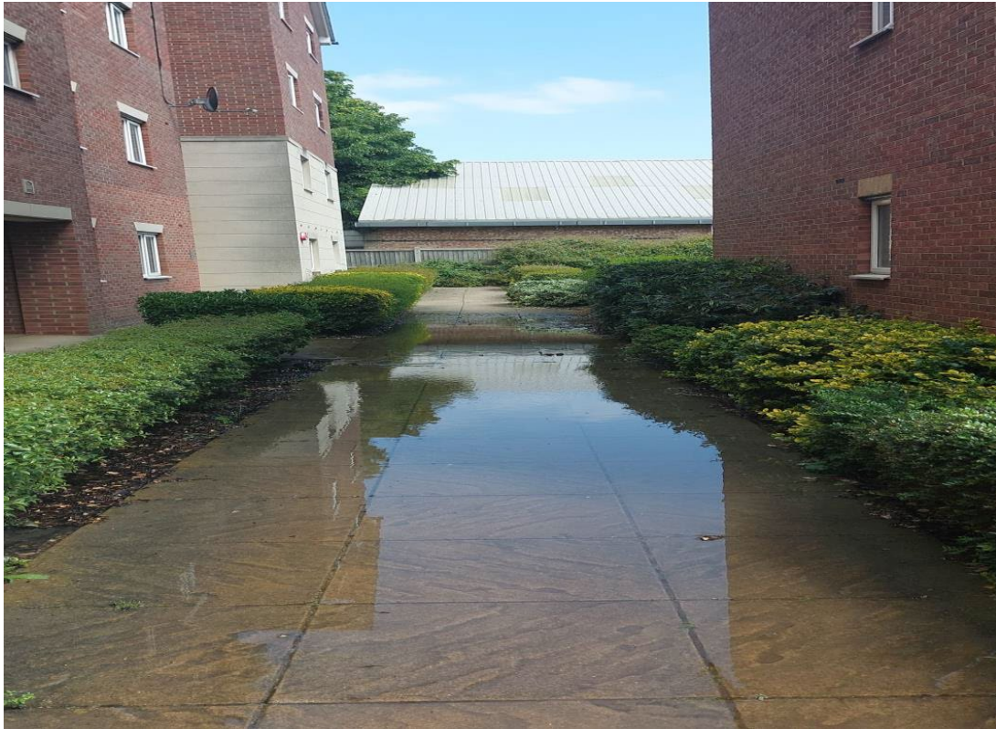
Attended site for flooded path/gardens
