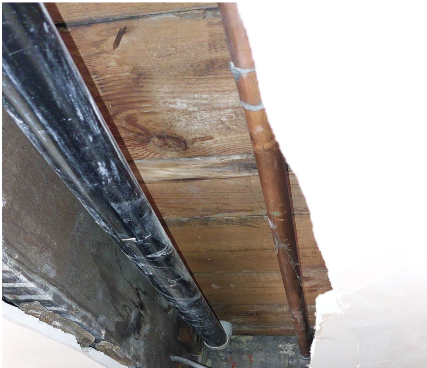
Replaced damage pipe work
