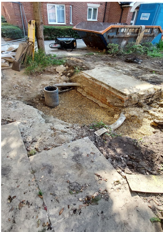
Ground bacfilled with compacted aggregates
