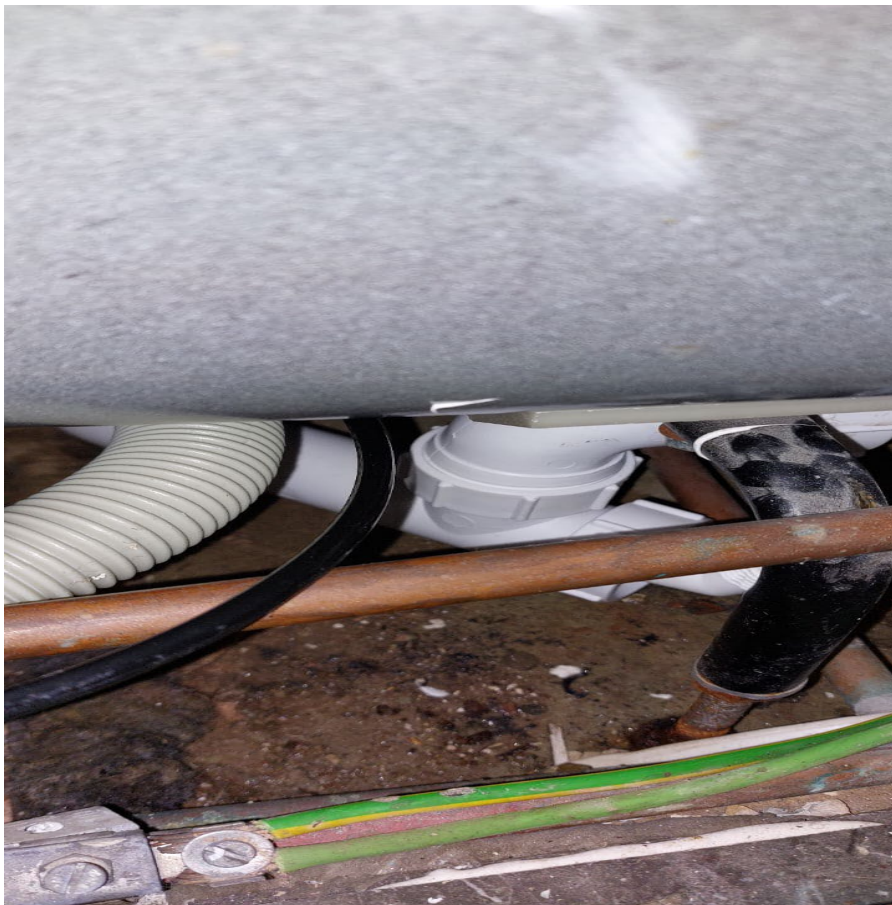
New plug waste kit fitted
