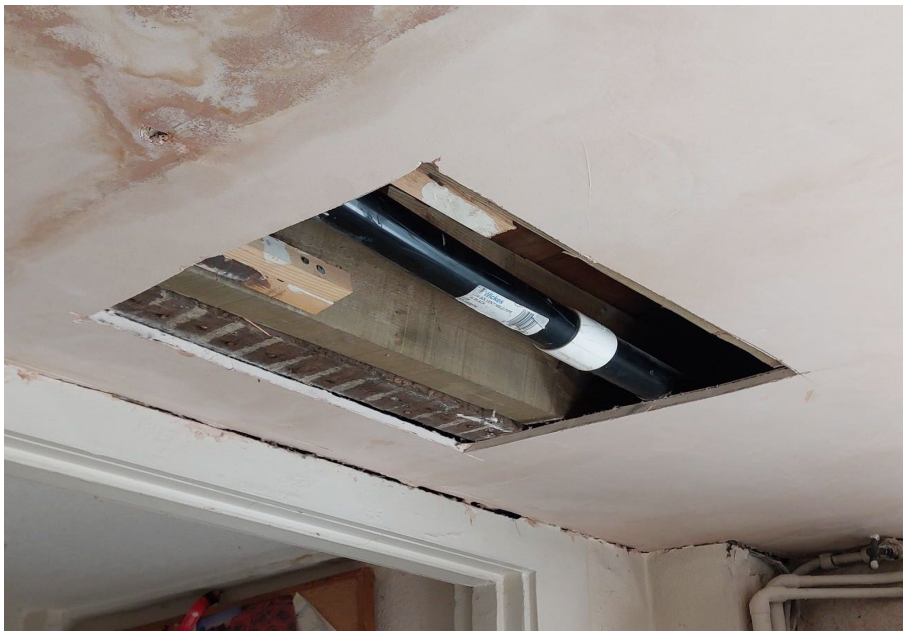
Pipe work replaced and leak resolved
