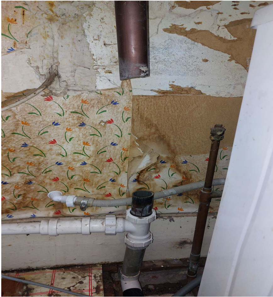
Removed the leaking pipe work
