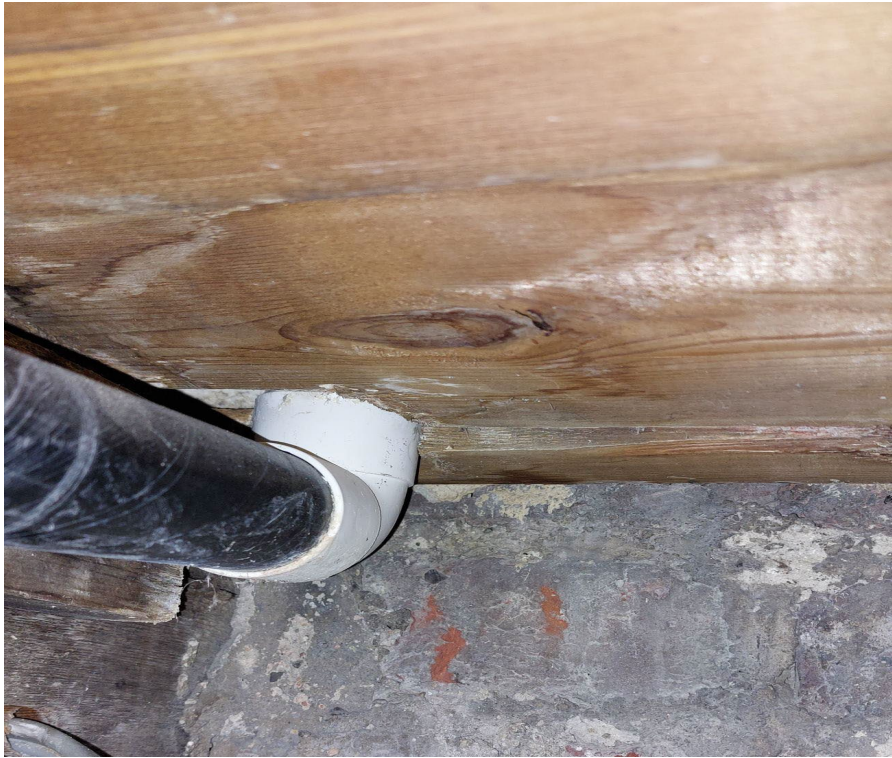
Replaced damage pipe work
