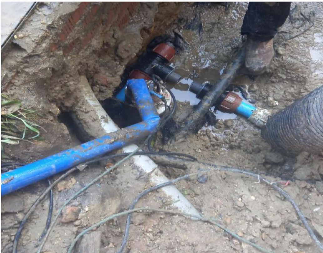
Supplied and fitted new fittings to repair the cold water supply pipe
