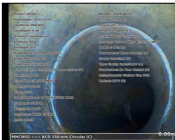
20260203-133243-snap0000.jpg, 00:00:03, 0.00 m Start node, manhole, reference: MHCW02
