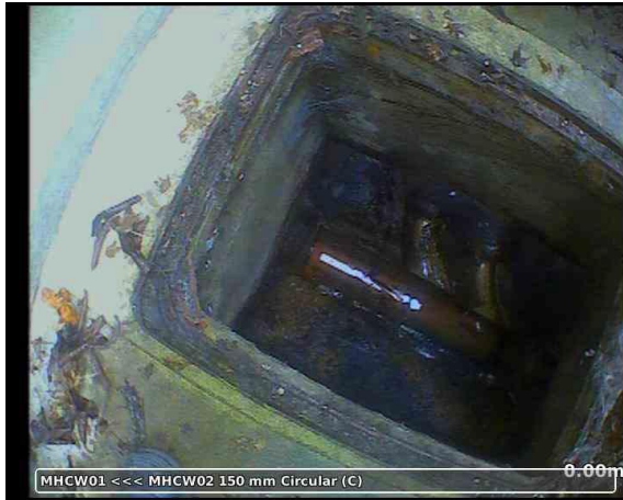
20260203-130158-snap0000.jpg, 00:00:03, 0.00 m Start node, manhole, reference: MHCW01
