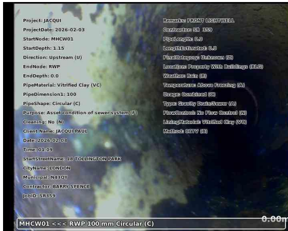
20260203-130931-snap0000.jpg, 00:00:03, 0.00 m Start node, manhole, reference: MHCW01
