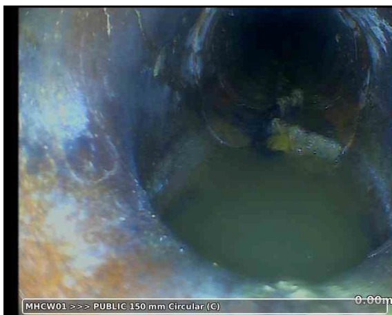
20260203-131500-snap0002.jpg, 00:00:22, 0.00 m Line deviates down, INTERCEPTOR
