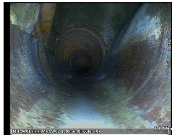
20260203-130158-snap0011.jpg, 00:05:49, 11.59 m Finish node, manhole, reference: MHCW02
