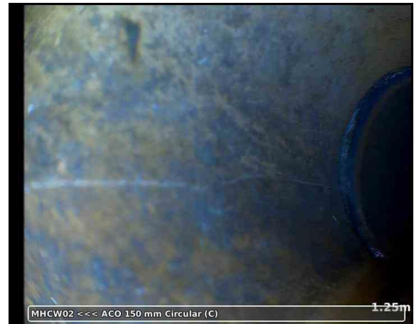
20260203-133243-snap0005.jpg, 00:01:21, 1.25 m Pipe size changes, new size(s), 100mm high
