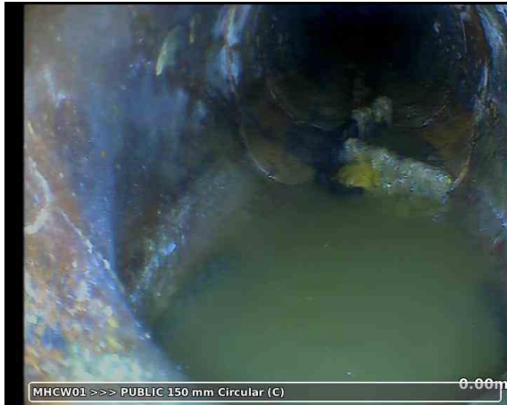
20260203-131500-snap0000.jpg, 00:00:06, 0.00 m Start node, manhole, reference: MHCW01
