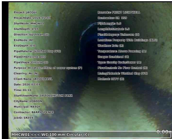
20260203-131157-snap0000.jpg, 00:00:02, 0.00 m Start node, manhole, reference: MHCW01
