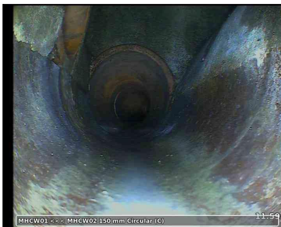
20260203-130158-snap0010.jpg, 00:05:41, 11.59 m Finish node, manhole, reference: MHCW02
