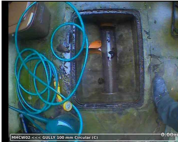
20260203-133026-snap0000.jpg, 00:00:03, 0.00 m Start node, manhole, reference: MHCW02
